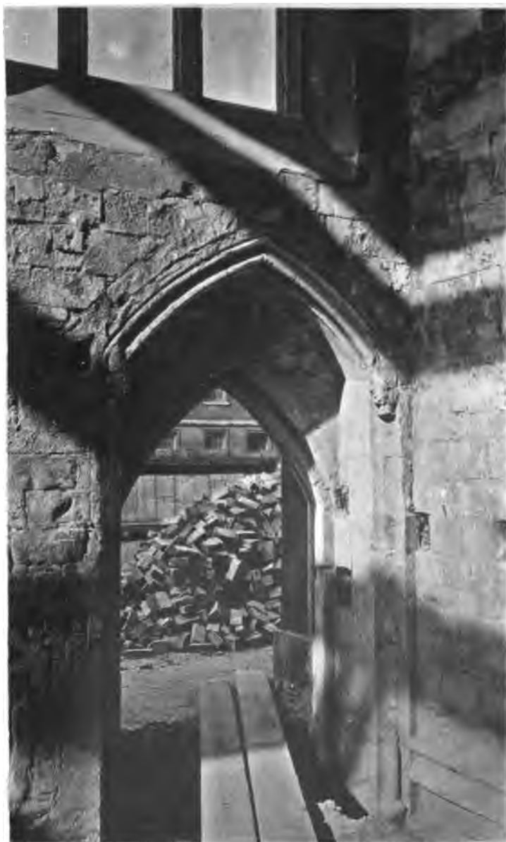
DOORWAY IN SOUTH WALL OF QUIRE. INTERIOR VIEW.
